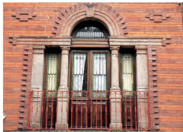
Detail of a facade on Serapio Rendón Street.
