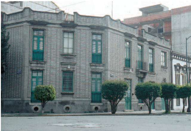
The neighborhood continues to be basically residential.
