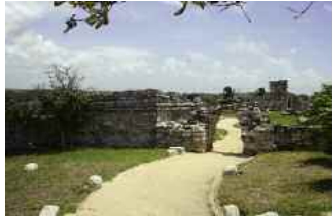
Access to the Interior Area, surrounded by a second wall.
