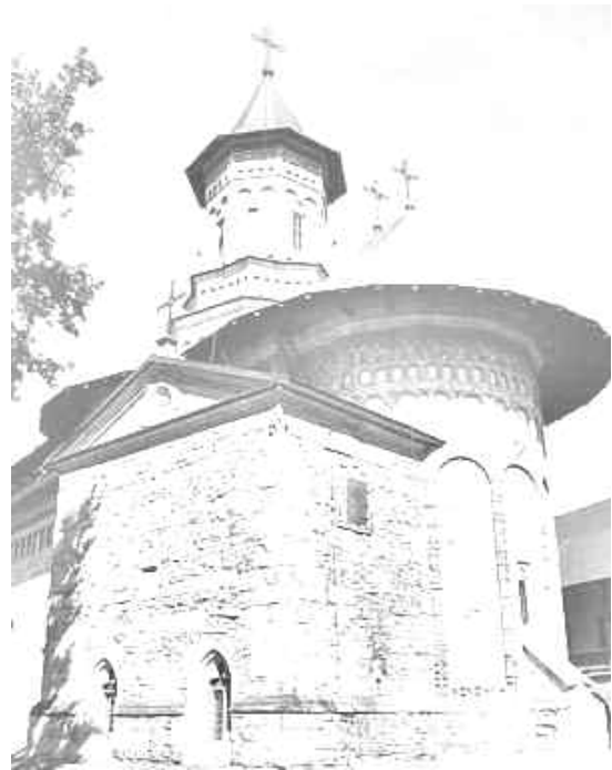
Neamt Monastery, Romania.
