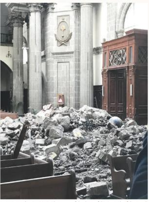
On September 24, 2017, a large part of the dome of the Our Lady of the Angels Church collapsed, depositing several tons of material inside the building.
