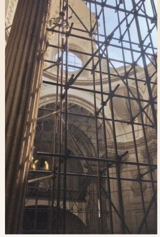
The interior arches of the Our Lady of the Angels Church next to the damaged area were protected: they are resting on a metal structure.
