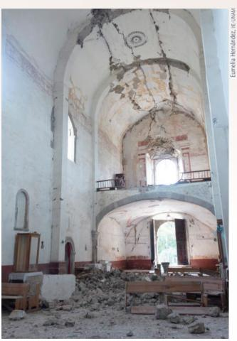
▲ Cracks and debris in the vault of the San Juan Bautista Church in Tlayacapan.
