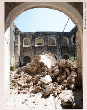
Debris from the collapse of the west gallery of the upper cloister in Totolapan.
