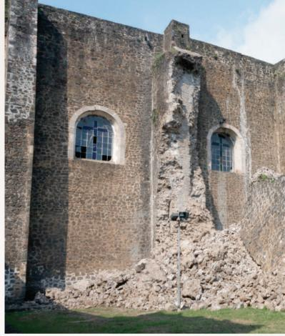
Collapsed buttress on the south side of the former Tlayacapan Monastery's atrium.
