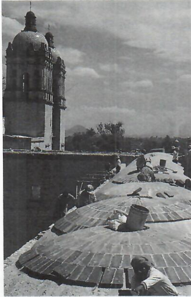
The restoration process.
