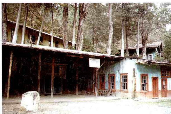
Part of the now-abandoned Dos Estrellas Mine offices.
