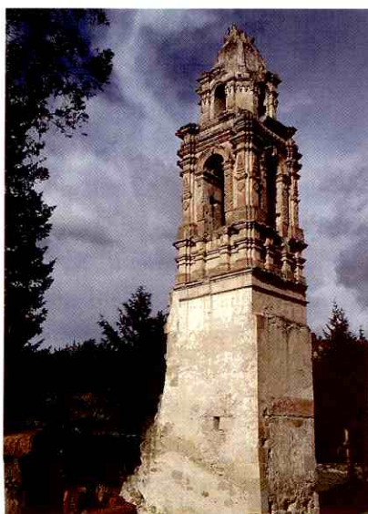
The bell tower of the old Our Lady of Carmen Church, left standing after the 1937 tragedy.
