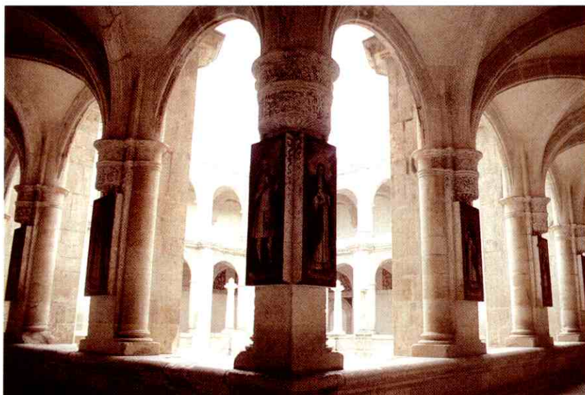
Construction techniques from the sixteenth century were recovered to restore the building's original appearance.
