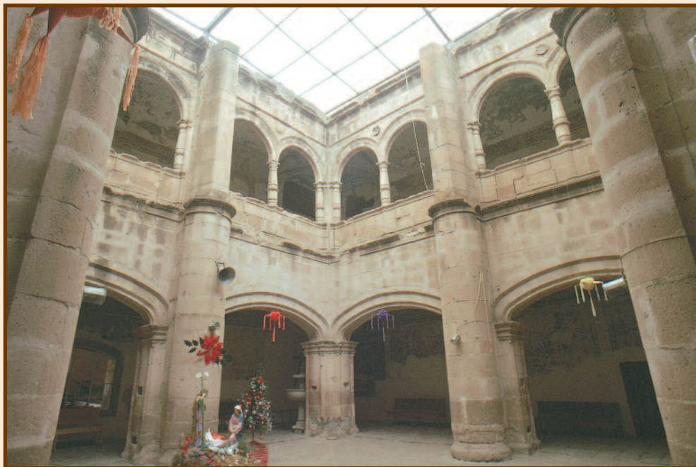
Corner of the cloister, Santiago Monastery, Copándaro.
